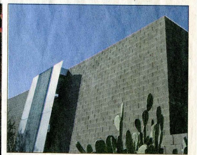
Top: A "desert modern" home built in 2001 and designed by Wendell Burnette is in the northeast Valley. Above: Will Bruder's design of Temple Kol Ami, at 64th Street and Greenway, is another Jarson favorite.
